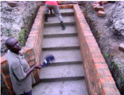
Picture 6. 3:Spring construction in Oyam
