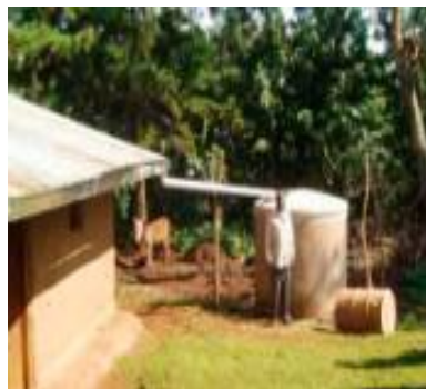
Picture 6. 12: Ferrocement Tank (4m 3 ) in Kapchorwa
