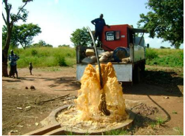
Picture 5. 6: Borehole blowing/cleaning in Pader
