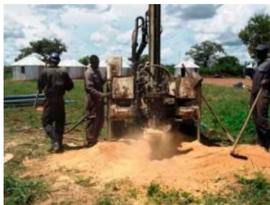
Picture 6. 7: Air percussion drilling with a light PAT 401 rig in Nwoya district
