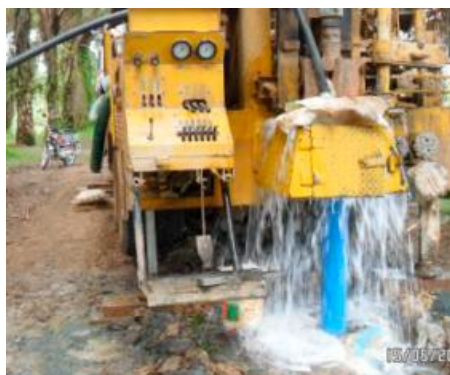
Picture 6. 8: Borehole development
