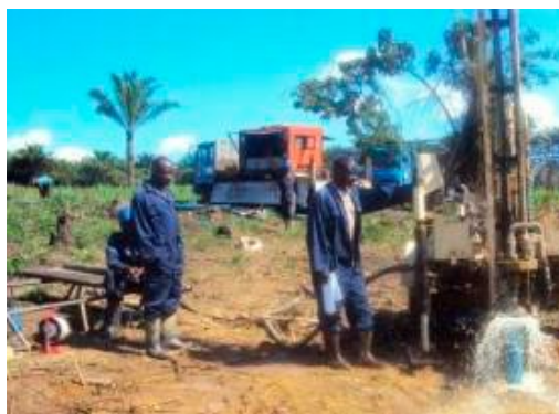
Picture 6. 9: Borehole drilling and development with a PAT 301 rig and an ELG 15 bar compressor
