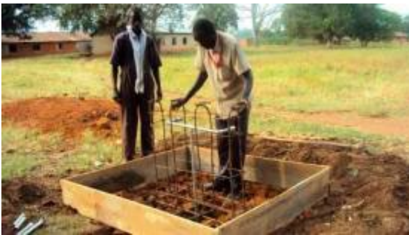
Picture 6. 16: Tap Stand construction in Oyam
