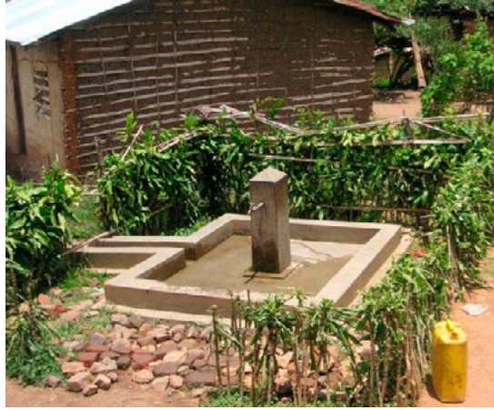
Figure 8. 1: A Well constructed and maintained tap stand in Kabarole
